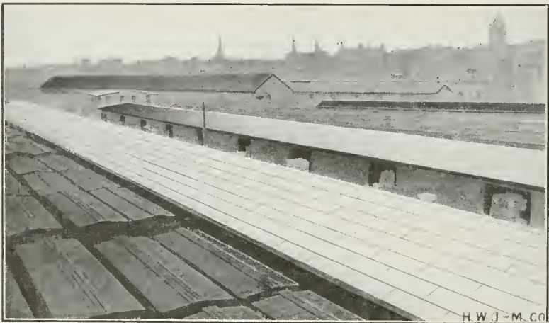
FIG. 71.—Freight sheds of the Boston and Maine railway, Boston, Mass. (Covered with asbestos slates.)
